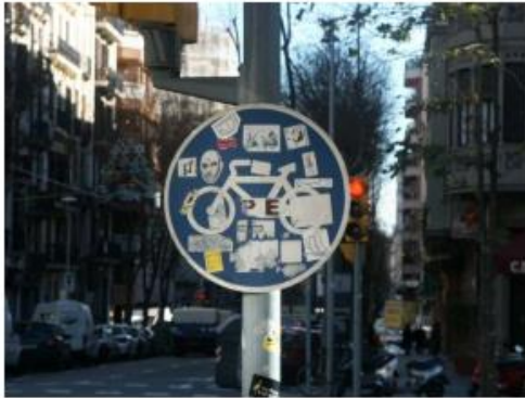
Figure 8. Stickers which damaged the pictogram of a sign.
